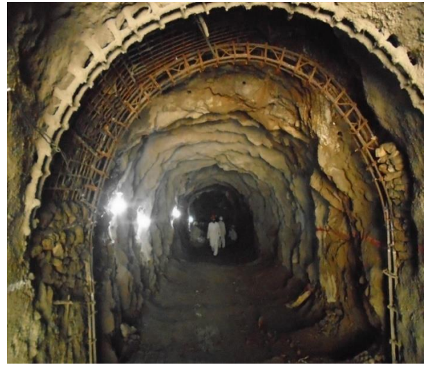
Figure 2 Tunnel construction at Karora [43].
